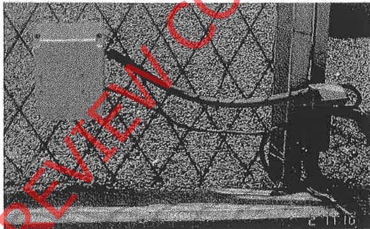
Figure 8. The enclosure mounted in parallel to the Sparkgap, which can be located near the gate to the high voltage yard.
