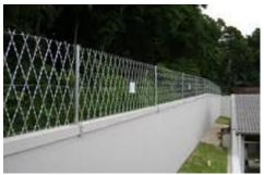
A Razor Mesh fence consists of straight blade netting welded together forming a diamond shape throughout the fence. Razor Mesh is a high quality product offering sufficient security for any property. Security can be further enhanced via an electrified wall top fence line.
